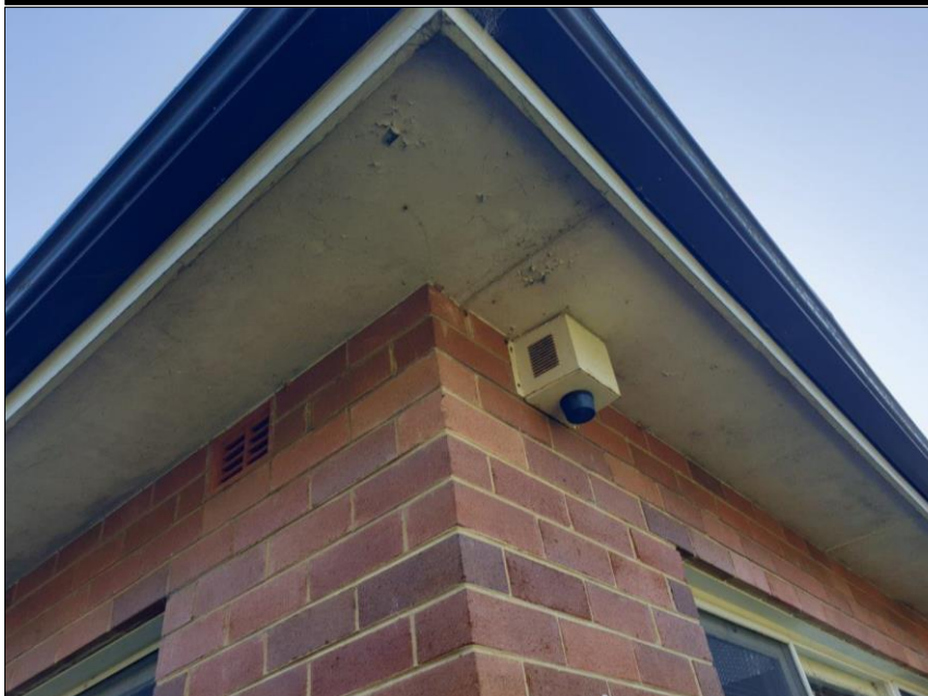
PHOTOGRAPH 16: 11 FIG TREE STREET – EAVES WITH POTENTIAL LEAD PAINT AND ACM
