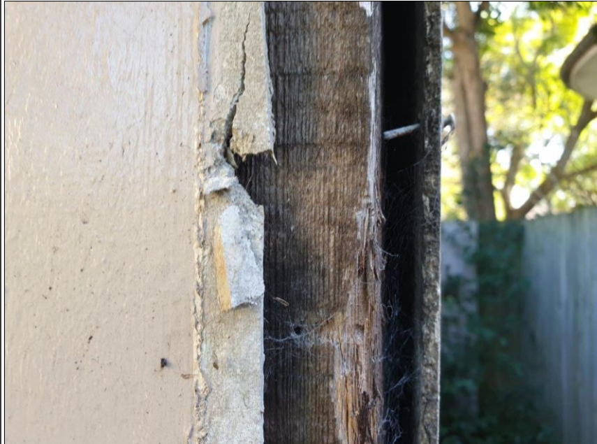
PHOTOGRAPH 44: 112 CENTENNIAL AVE - DAMAGE TO POTENTIAL ACM SHEETING PRESENT ON GARAGE
